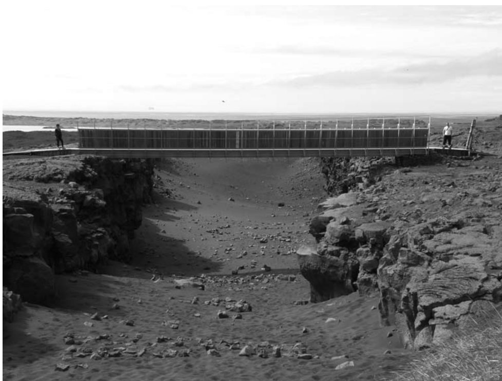
FIG. 11. The "Bridge Between Two Continents", Iceland: left – North America; right – Europe.
